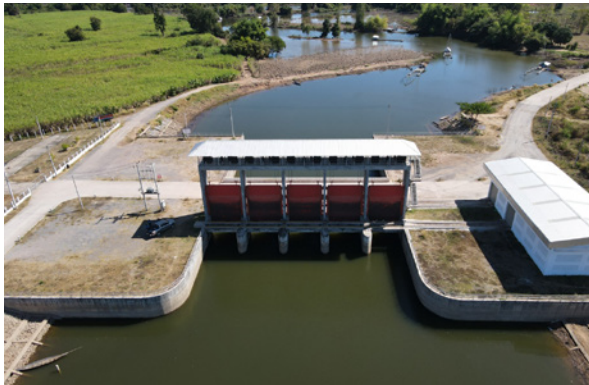
Large-scale Irrigation Project: Nam Churn Watergate, Ban Kut Khaen, Nong Ruea District, Khon Kaen Province
