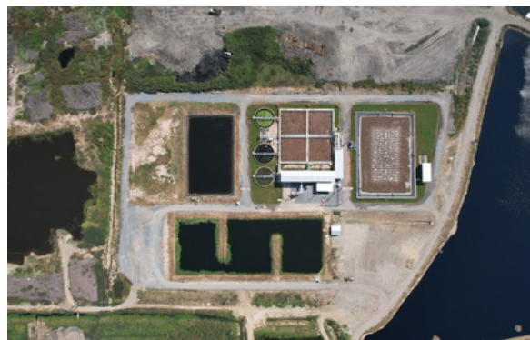
Activated Sludge System in the area of Dan Chang Complex
