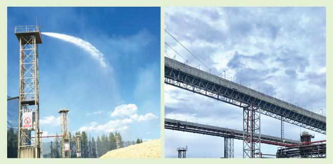
Controlling dust at bagasse storage facilities by spraying water and installing conveyor belt covers.
