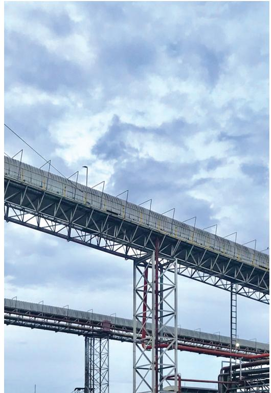
*Controlling dust from bagasse storage areas such as using the water spray to prevent diffusion of bagasse and installing the cover of the bagasse conveyor bridge.*
